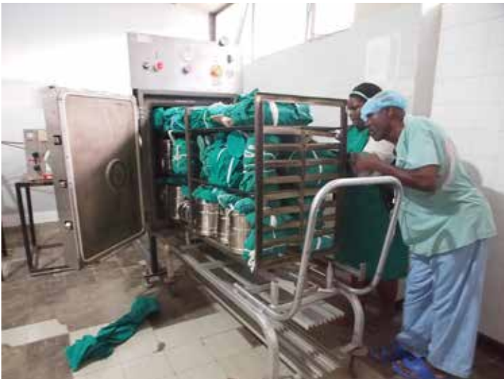
Fig. 5: Loading one of the two autoclaves based on the AmSCO Medallion at the Bugando Medical Centre, Tanzania (29.11.2019).
