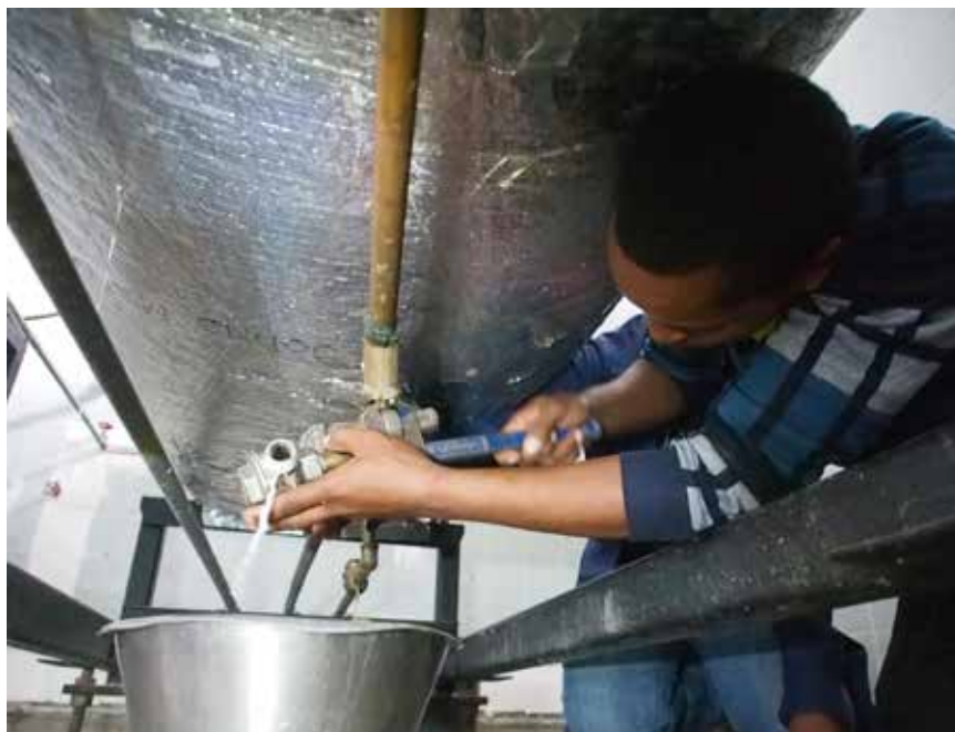
Fig. 8: A technician removes the steam trap that turned out to be defective (04.12.2019).
